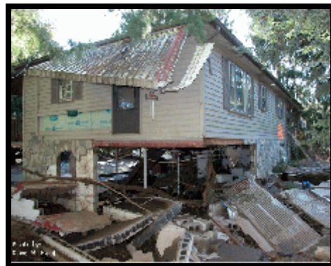
A destroyed home in Haywood Co., NC.
