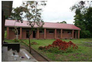
Two class rooms and a multipurpose room.
