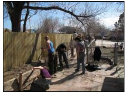
Building Auntie Mary Ann's fence.
